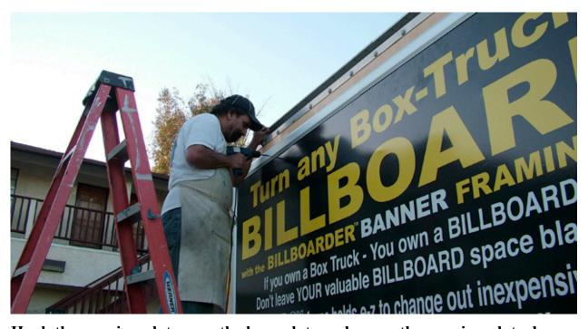
Hook the capping plate over the base plate and screw the capping plate down onto the base plate utilizing the self tapping screws a foot apart and into and along the screw groove on the capping plate, which will tighten the banner further.
